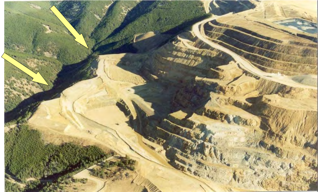
Swift Gulch Drainage, 2001. BLM Photo.
