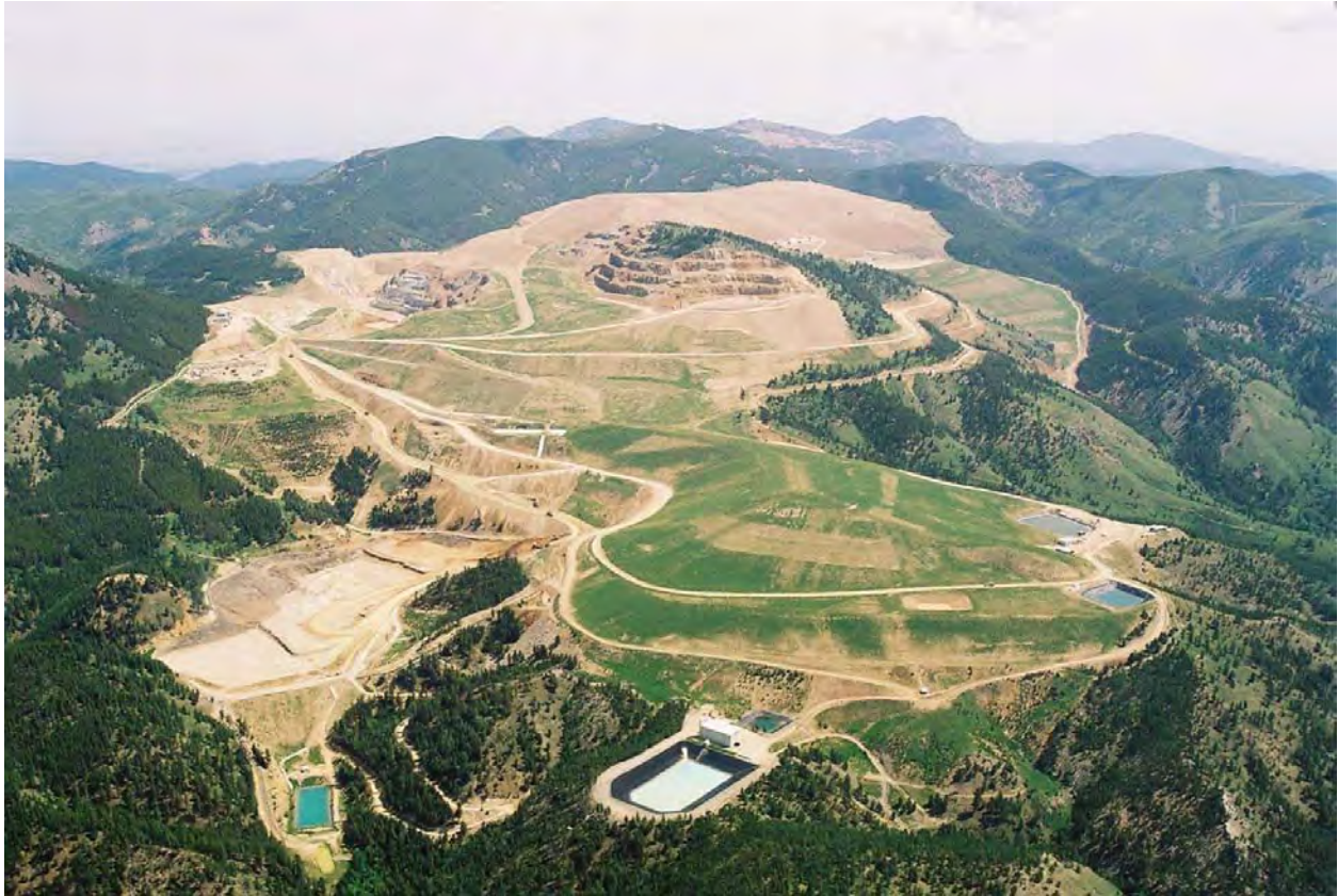
Landusky Water Treatment Plant, 2004. BLM Photo.
