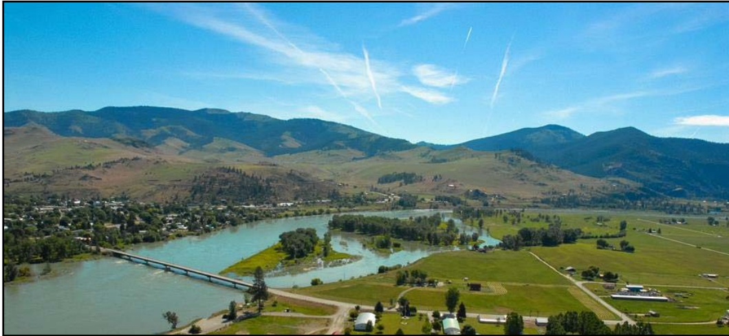
Sanders County received a Watershed Planning Grant to evaluate alternative solutions to bank erosion on the Clark Fork River upstream from the Plains Wastewater Treatment Plant. High sediment loads also adversely affect fish habitat and reservoir capacity.
