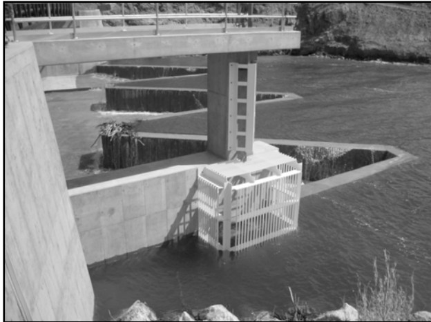
New Labyrinth Weir Above Ruby Dam Spillway
