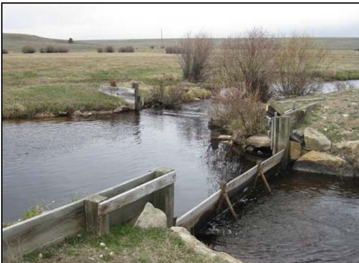
The Beaverhead County Conservation District received a Renewable Resource Project Grant to construct a siphon across Swamp Creek located near Wisdom. The Siphon will replace a diversion structure allowing water users more flow control and restoring connectivity to the Big Hole River for fish passage.
