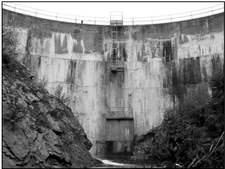
Flower Creek Dam Replacement Project Renewable Resource Grant to the City of Libby
