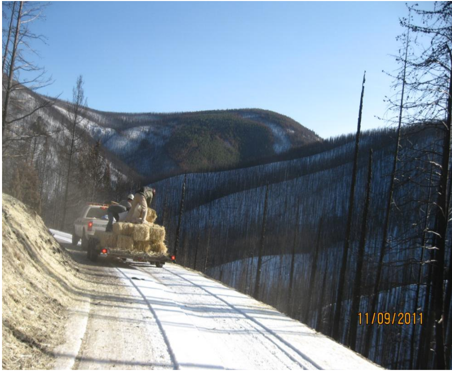
Figure 4. Straw mulch and seed being applied to stabilize roads within the burned areas.
