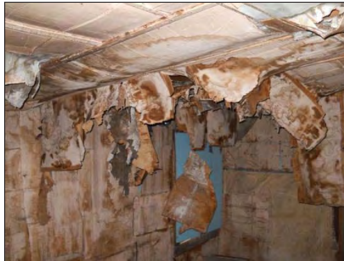
No south interior wall remains in the Cogswell Cabin to shelter it from the elements, and the protective muslin is clearly beyond repair with weather and water damage.
