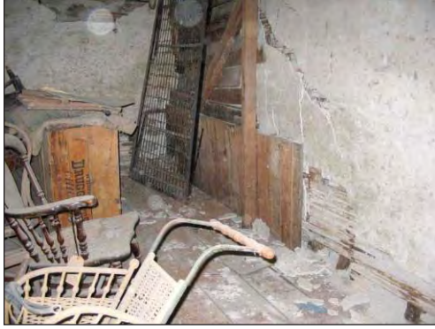
The Wells Fargo Office has major interior damage to the historic lath and plaster, and the exterior needs oiling
