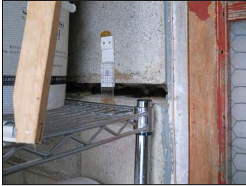
Figure 12: Crack monitor on the rear façade of the City Bakery shows the growing displacement of the building at an alarming rate.
