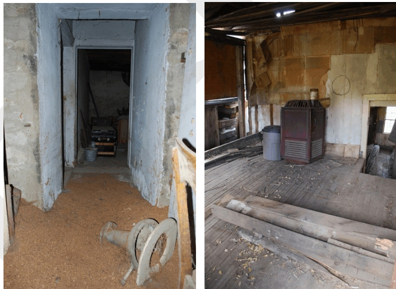
Examples of preservation work needed in Virginia City. At left: The back of the E.L.Smith Store. At right: Cogswell Cabin where the log wall on the left has rotted away. Photos by Hope Stockwell
