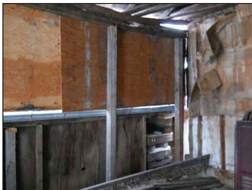
No south interior wall remains in the Cogswell Cabin to shelter it from the elements, and the protective muslin is clearly beyond repair with weather and water damage.
