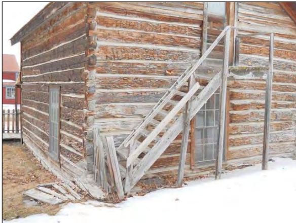
Figure 15: Rotting boards require consolidant
