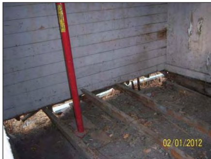
The interior of an addition to the Hickman House sitting on floor joists exposed to the element, interior decay
