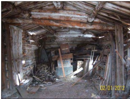
The George Ives Jail: an original Nevada City structure in danger of collapsing. Bottom right: an archaeological test unit filled with ice is proof that the building needs regarding.
