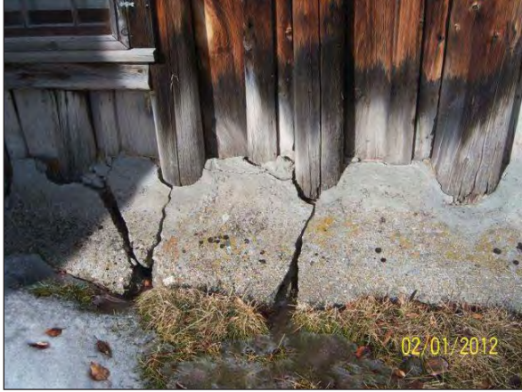
“Bovey Backfill” has failed, leaving cracks and spaces for moisture to accumulate, accelerating wood rot along the entire exterior of structure
