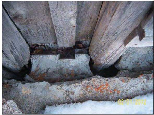
“Bovey Backfill” has failed, leaving cracks and spaces for moisture to accumulate, accelerating wood rot along the entire exterior of structure
