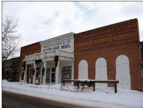
The brickwork on Virginia City's upscale restaurant, the Wells Fargo Coffee House, is in need of re-pointing
