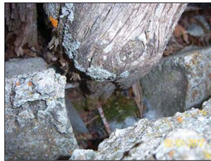
The Nevada City Hotel sits on large upright beams, some that do not even touch the ground (above right)
