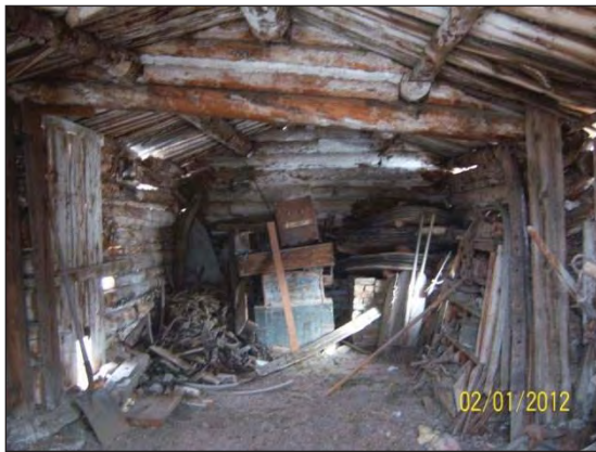
The George Ives Jail: an original Nevada City structure in danger of collapsing. Bottom right: an archaeological test unit filled with ice is proof that the building needs regarding.
