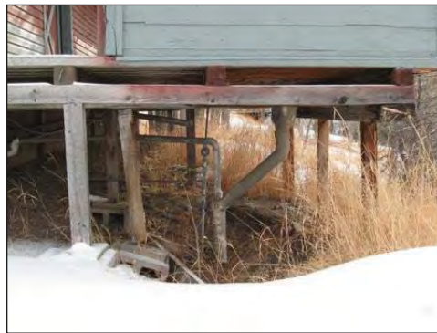
The Virginia City Depot bathrooms sit precariously at the corner of the porch with little structural support
