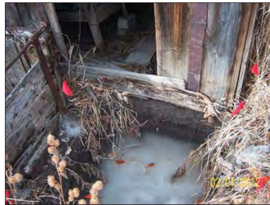
The George Ives Jail: an original Nevada City structure in danger of collapsing. Bottom right: an archaeological test unit filled with ice is proof that the building needs regarding.
