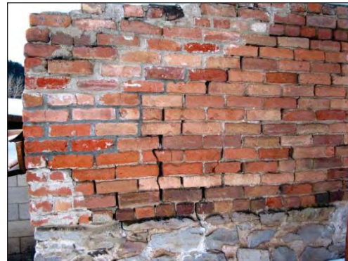
The brickwork on Virginia City's upscale restaurant, the Wells Fargo Coffee House, is in need of re-pointing
