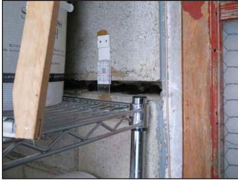
Figure 12: Crack monitor on the rear façade of the City Bakery shows the growing displacement of the building at an alarming rate.
