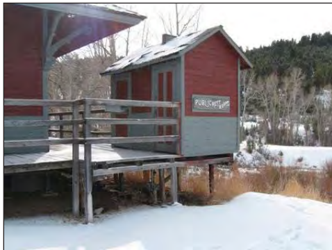
The Virginia City Depot bathrooms sit precariously at the corner of the porch with little structural support
