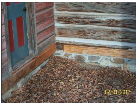
Preserved building has new foundation and sill logs
